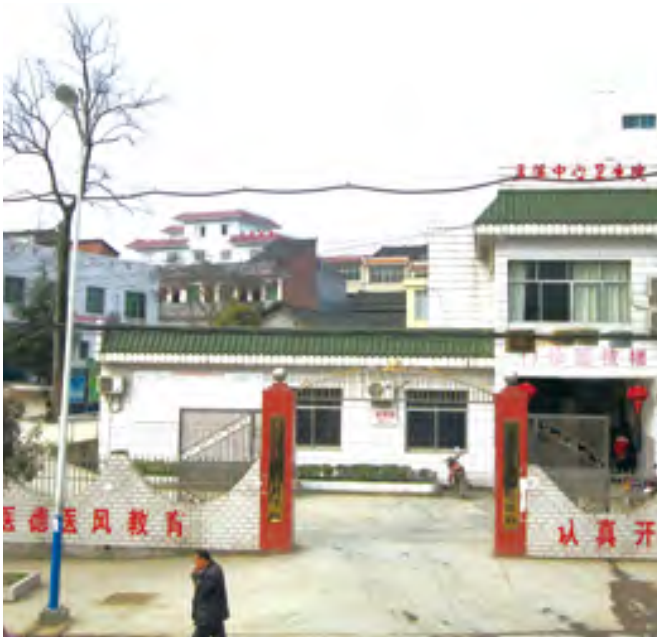
修建前 Central Health Institute before renovation ( photo )
