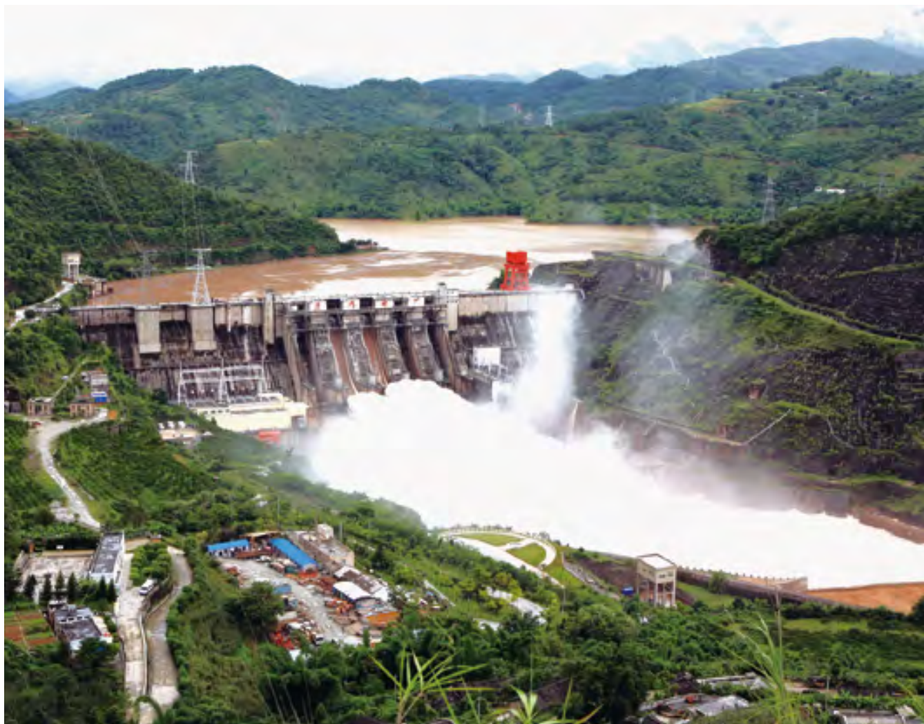
澜沧江漫湾电站 Manwan Hydropower Station on the Lancang River
