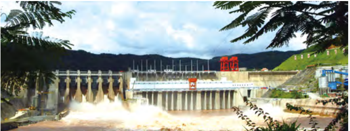
澜沧江景洪电站 Lancangjiang Jinghong Power Station
